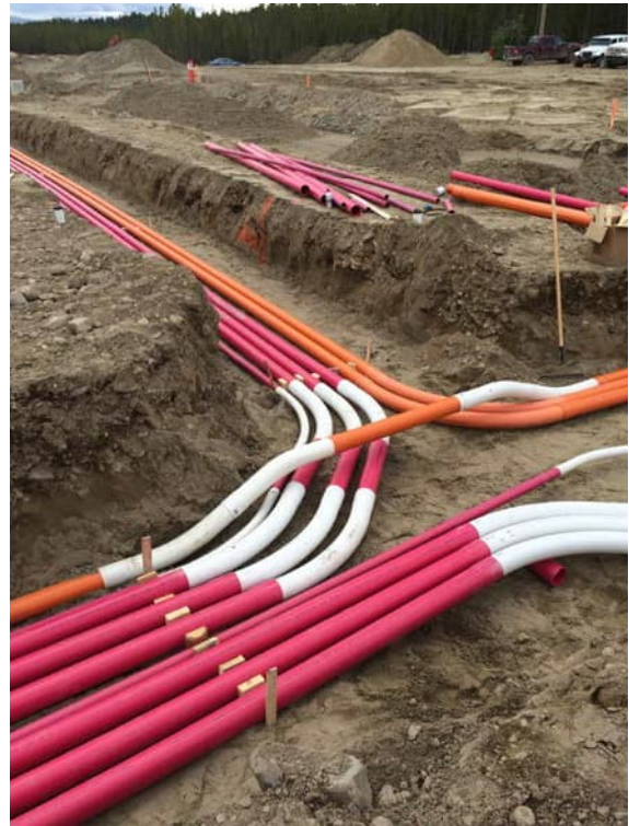
Note how orange conduits are placed to allow pedestal entry minimizing crossovers. Note also how they come out of the pedestal in a planned manner for the next site. Orange over red is the rule.
