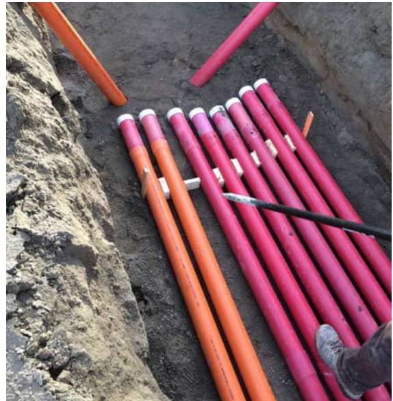
Note: When ducts end on the straight end, you can use a cap. When ending on the bell end, use a short piece of conduit and a cap. Do not glue caps!
