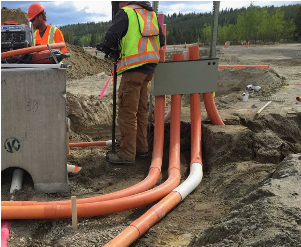
Note how the sand mound is carved away to allow duct entry
