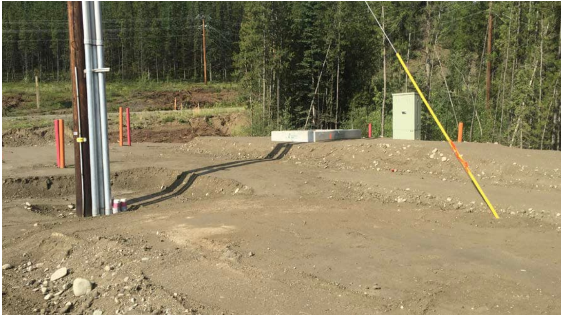
Proper vault and TV2500 setting elevations
