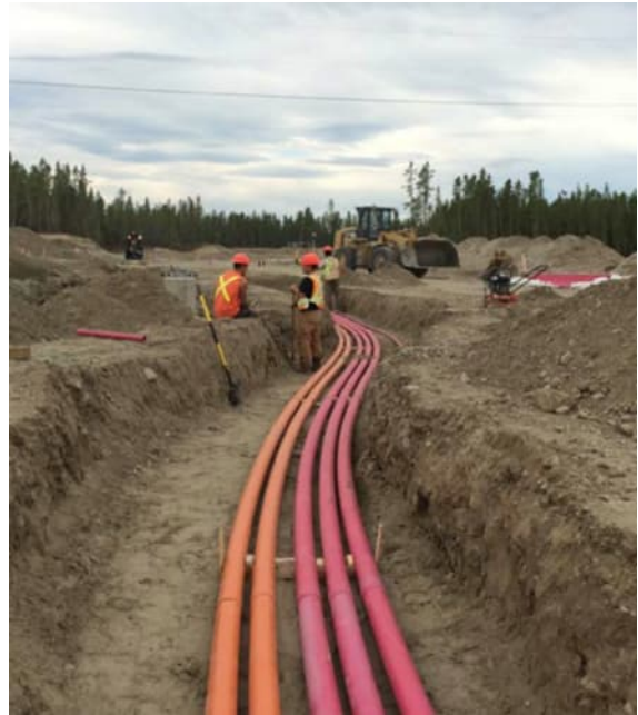
Note conduits curved and staked in place.
