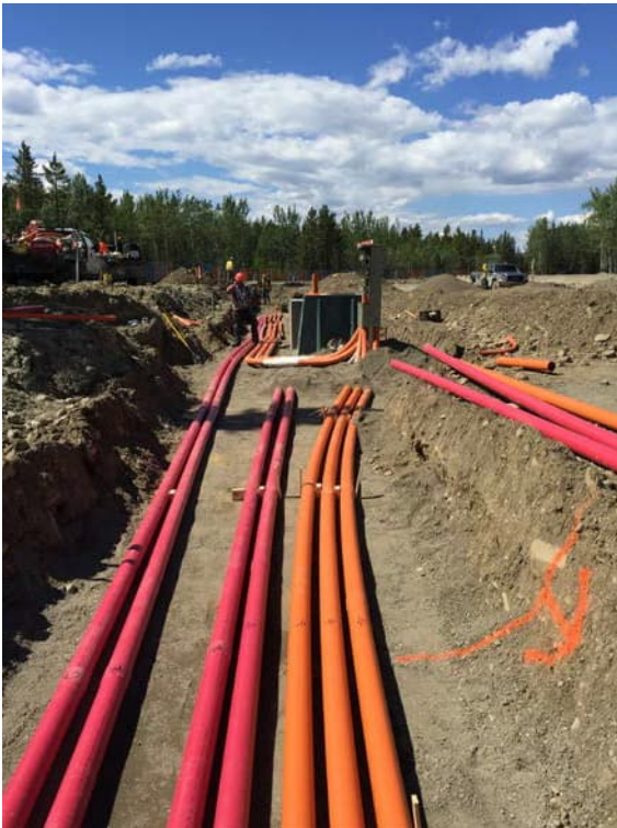
Note how orange conduits are placed to allow pedestal entry minimizing crossovers. Note also how they come out of the pedestal in a planned manner for the next site. Orange over red is the rule.
