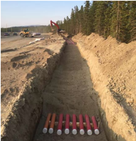
Note: When ducts end on the straight end, you can use a cap. When ending on the bell end, use a short piece of conduit and a cap. Do not glue caps!
